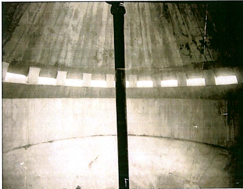
Above: Imhoff Tank from directly above 1913; Below: Interior Sludge Digestion Chamber 1913 [City of Kelowna]
