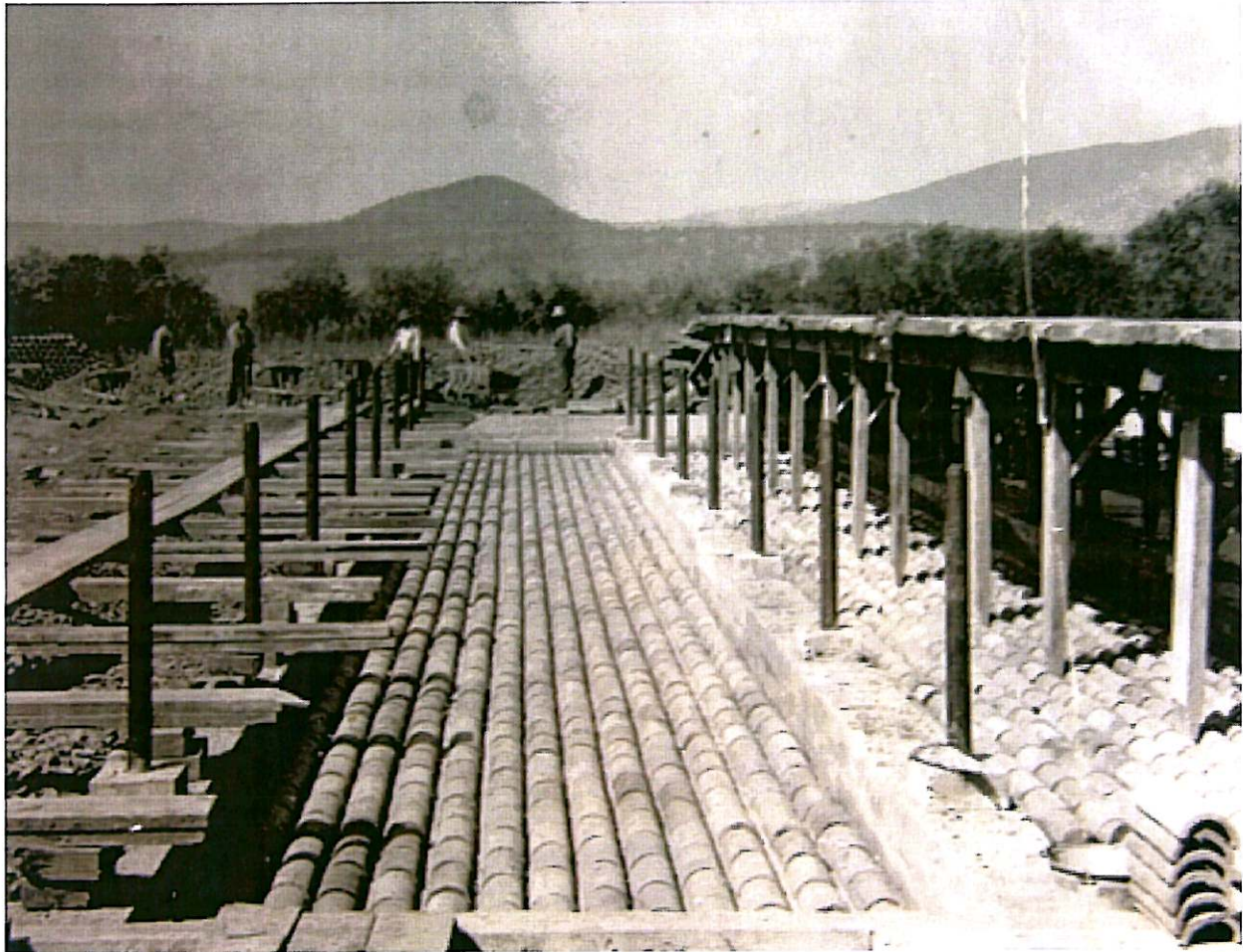
Above: Filter during Construction 1913; Below: Dosing Tank discharging on Sprinkler Filter 1913 [City of Kelowna]
